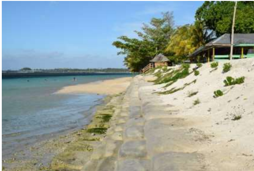
Figure 38: Example use of Sand bags on regraded beach profile with associated vegetation planting
