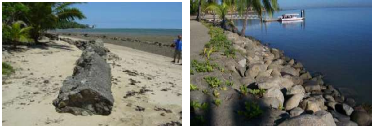
Figure 36: Seawalls as Hard measures are known to be ‘brittle’ options that require much assessment and tailored design to ensure effectiveness. They will protect assets behind the wall but will often cause more sand erosion along the beach
