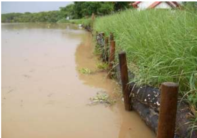
Figure 25: After 12 months the Vetiver grass stabilizes the banks
