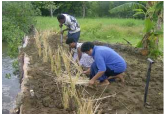
Figure 24: Backfilling behind the natural log wall and planting of Vetiver grass
