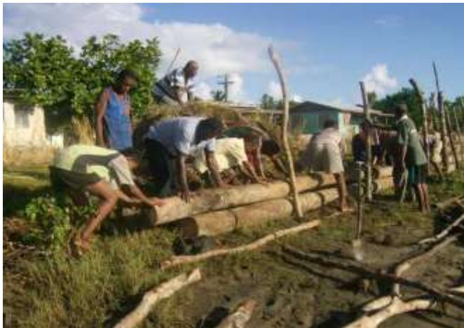
Figure 23: Community using local materials to stabilize the river bank
