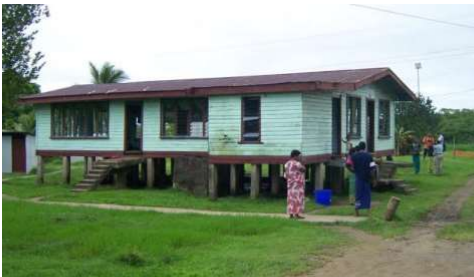
Figure 20: Existing wooden substantial buildings can be lifted from concrete foundations onto piers
